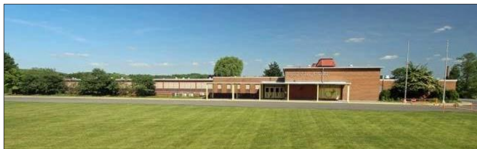
Gilbert Linkous Elementary – replace front fence, replace concrete sidewalks, construct canopy, and conversion of classrooms.
