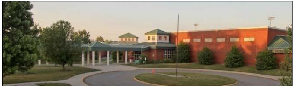
Auburn Elementary – replace bathroom floors
