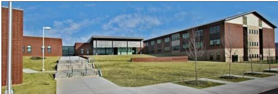
Blacksburg High – install field irrigation, develop a plan for locker rooms, concession stand, seating, and restrooms for baseball and softball.
